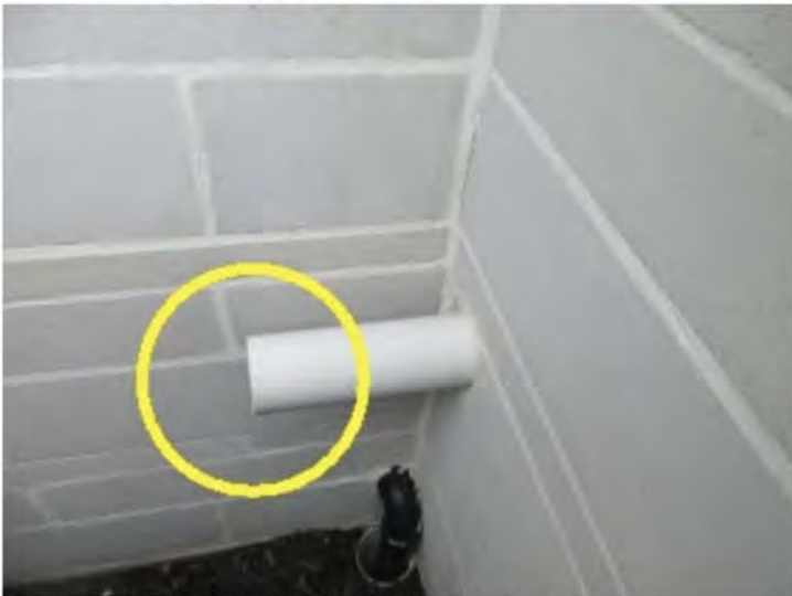
Scupper (flat roof drain)
