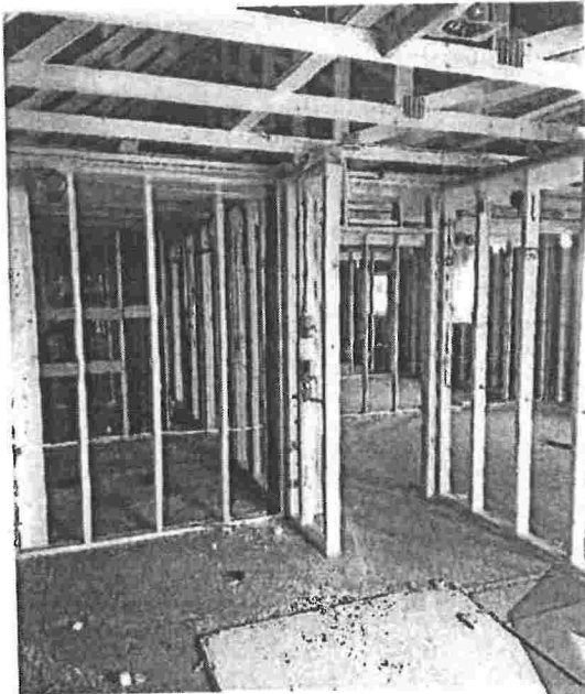
Figure 68 Building 11 Interior framing
