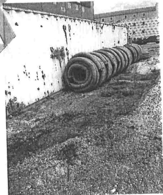
Figure 75 Weeping tiles on laydown
