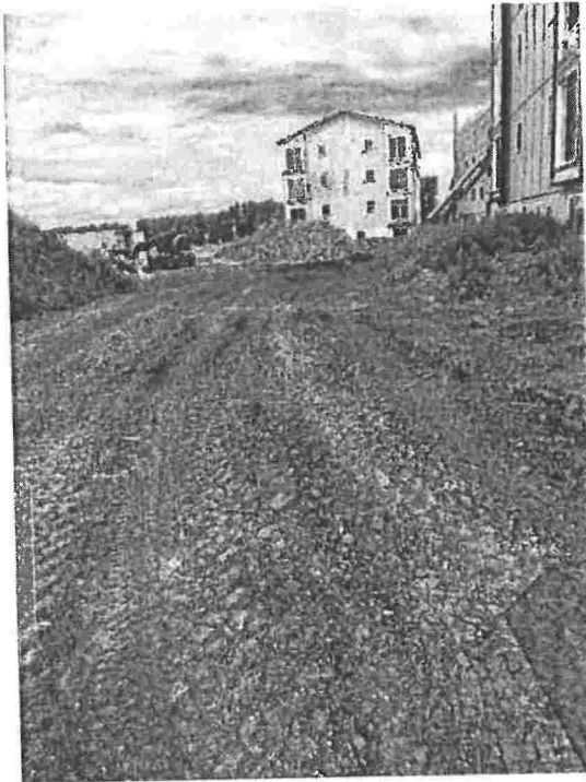
Figure 76 Parking lot on west grading
