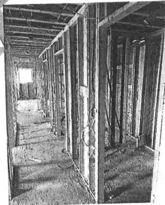
Figure 67 Building 10 Electrical Rough Ins
