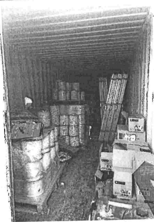
Figure 72 Electrical materials in storage
