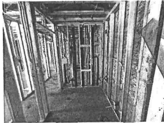
Figure 14 Building 1 Typical Rough ins
