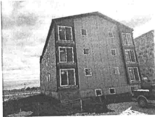
Figure 7 Building 1 -West Elevation
