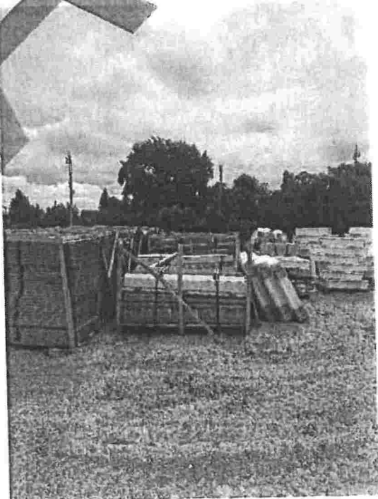
Figure 71 HM steel door and frame laydown
